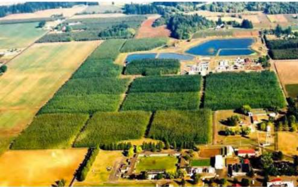
Precedent: Woodburn OR, Wastewater Treatment Facility Source: CH2MHill
